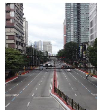
Figure 3.26 : Examples of medians from across the globe. (Left) Grill and kerb median on sub-arterial road. (Right) Landscaped median with crash barrier on arterial road.
