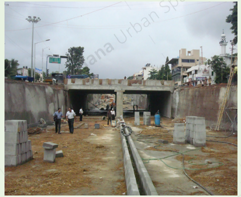
Image 2.22 >> Under Pass construction on Hosur Road, Bangalore using pre cast elements and soil nailing techniques
