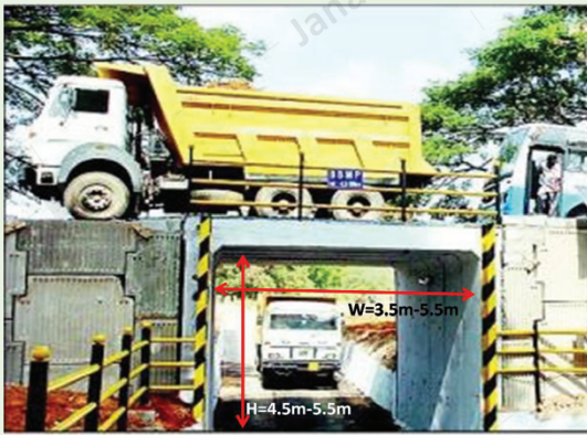
Image 2.21 >> Jacked Box Tunnelling (imagesource: http://indianrailways.informe.com/forum )
