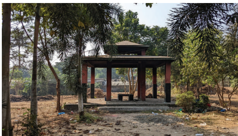
Figure 2. Existing crematorium shed in Bhubaneswar, Odisha
